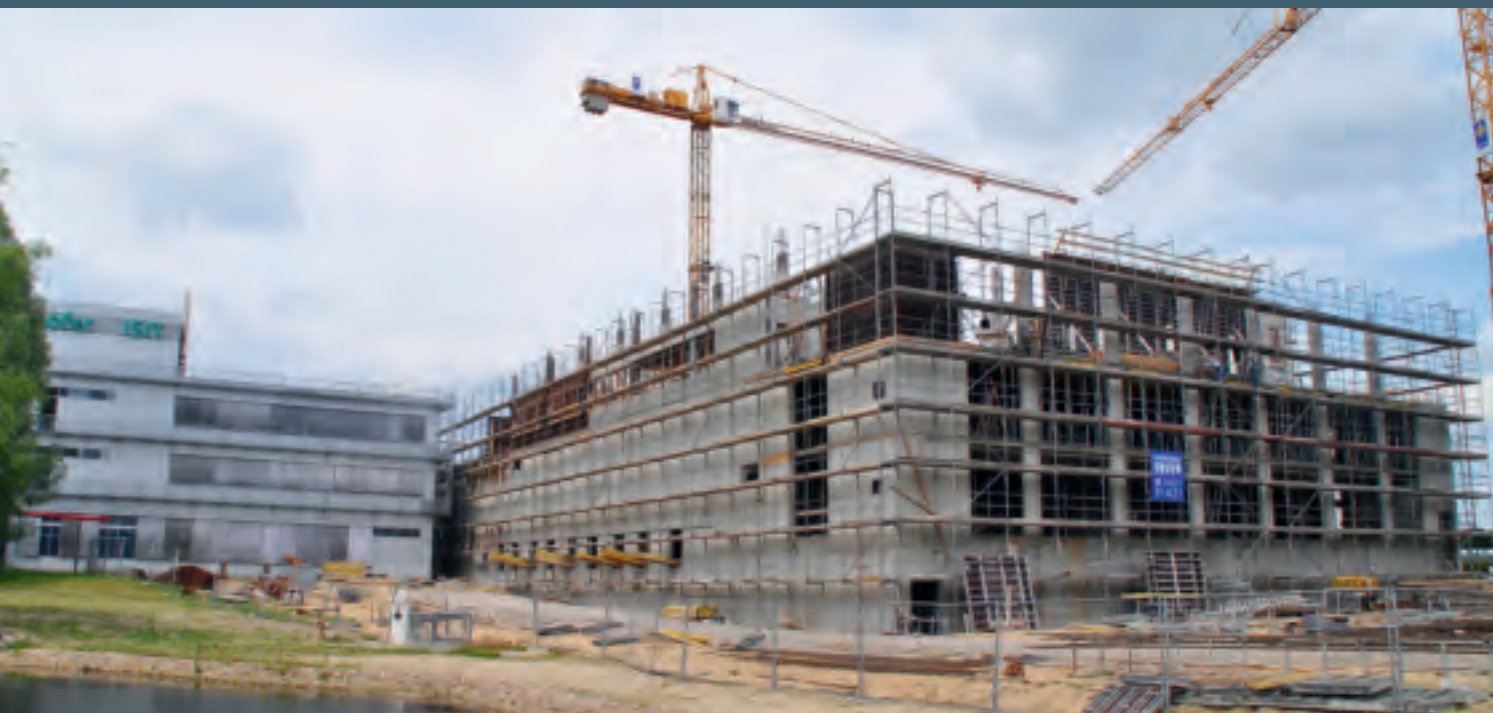
ISIT cleanroom building II under construction in 2012
